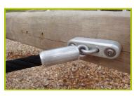
5- The fixings for the nets and chains are made from aluminium.
