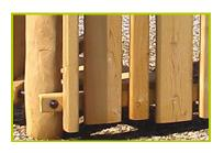
**2- The panels and the shelf** are made from larch (plank sizes 140 x 27mm / 45 x 68mm). Larch is naturally resistant and long lasting.
