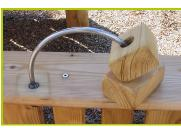
6- The abacus pieces are made from larch. The rail is made from 10mm diameter stainless steel.
