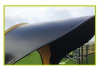
2- The roof is made of aluminium painted sheet.
