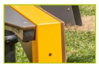
**5- The Central Column seating** is supported by a painted galvanized steel frame structure.
