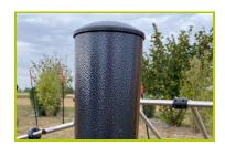
1- The 102mm diameter post is made of painted galvanised steel. The grained finish has a slightly undulating surface for increased scratch resistance. The cap is made of painted aluminium.
