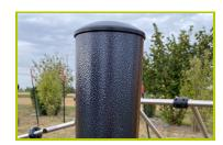
**1- The 102mm diameter posts** are made of painted galvanised steel. The grained finish has a slightly undulating surface for increased scratch resistance. The caps are made of painted aluminium.
