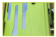
**6- The decorative fence panels** are made of 3mm thick painted aluminium sheets.
