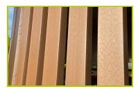
**4- The slatted fences** are made of composite wood (slats of 70 x 30 mm), which is a chip and split resistant waterproof material with UV protection.
