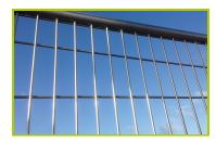
9- The panels are made of stainless steel mesh netting, Ø 6mm.
